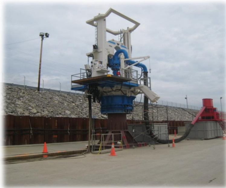
Photograph 4. Wirth pile top equipment drilling secant piles.
