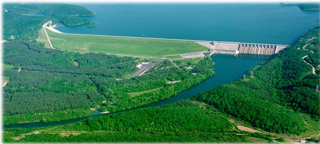
Photograph 1. View of Wolf Creek Dam, KY.
