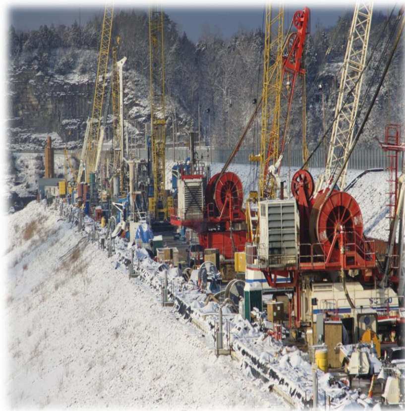
Photograph 6. View of Working Platform showing very congested conditions, including two hydromills.
