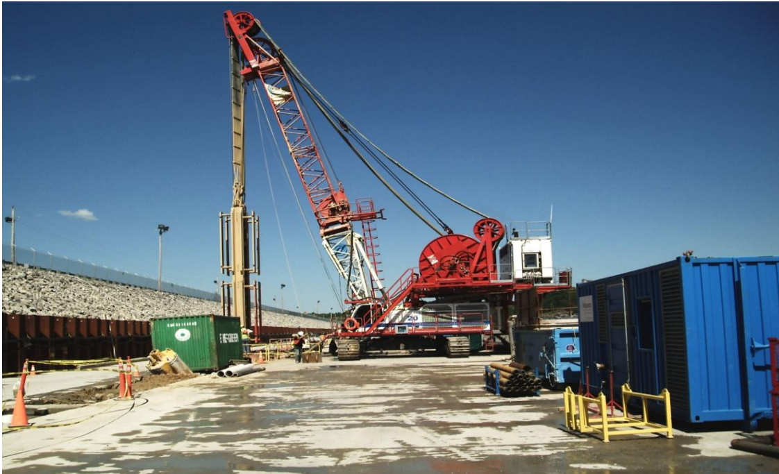
Photograph 5. New generation hydromill excavating 72-inch wide PCEW.
